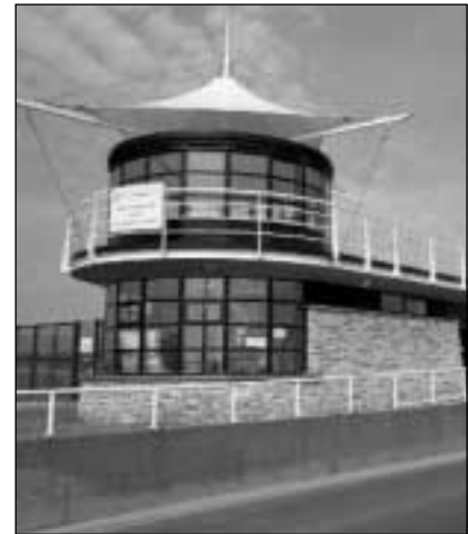
Hornsea Boat compound
